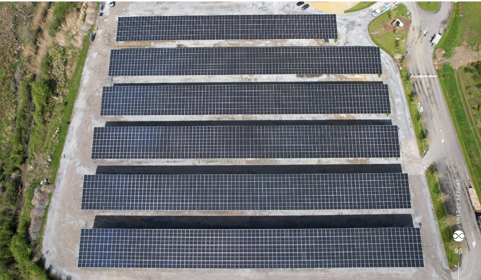
✓ The sustainable solar car park at Adventure Valley in Durbuy, featuring no less than 2,480 solar panels.
